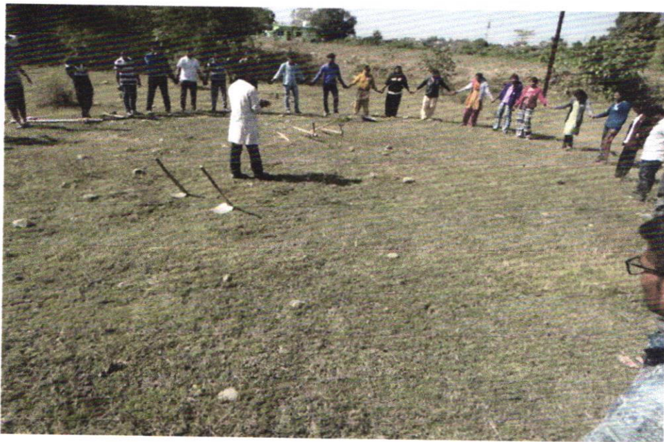
During the session 2017-18 the NSS Camp theme was “Environmental Awareness including preservation of natural resources and conservation of cultural /historical heritage”. The volunteers of NSS team constructed the “Bandara” over the local lake of the wadgoan village, tehsil Seloo. On the demand of the villagers and under the guidance of the engineer, working in “PANI FOUNDATION” team, our students constructed it with their hard work.
